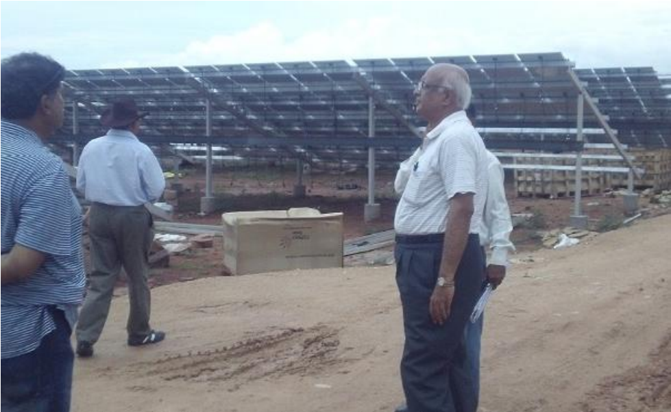
VTI Engineers on-site of a 5.5 MW Solar Power Plant at Bap, Rajasthan.
